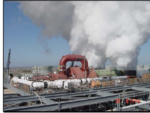
HV Steam Blow
