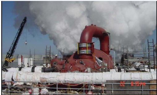
HV Steam Blow
